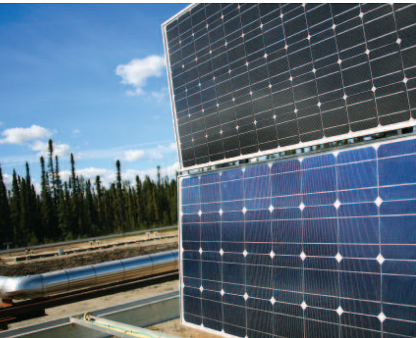
Solar panels are used to run the control systems (SCADA) on observation wells at our Christina Lake oilsands operations.
