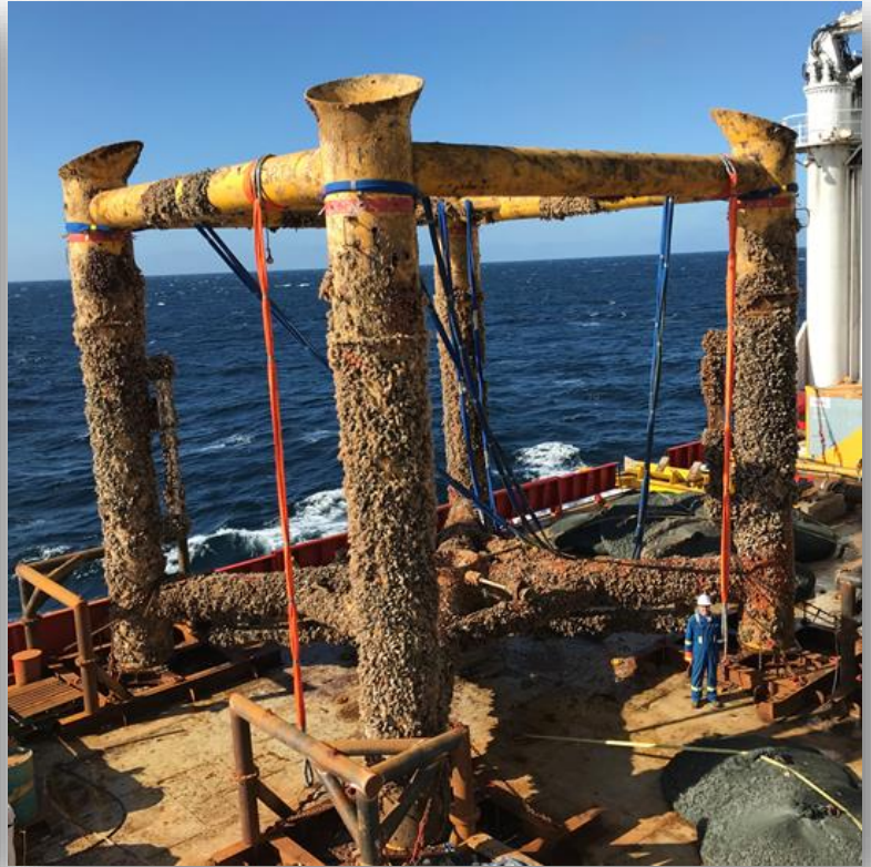
H-08 wellhead protection structure on deck
