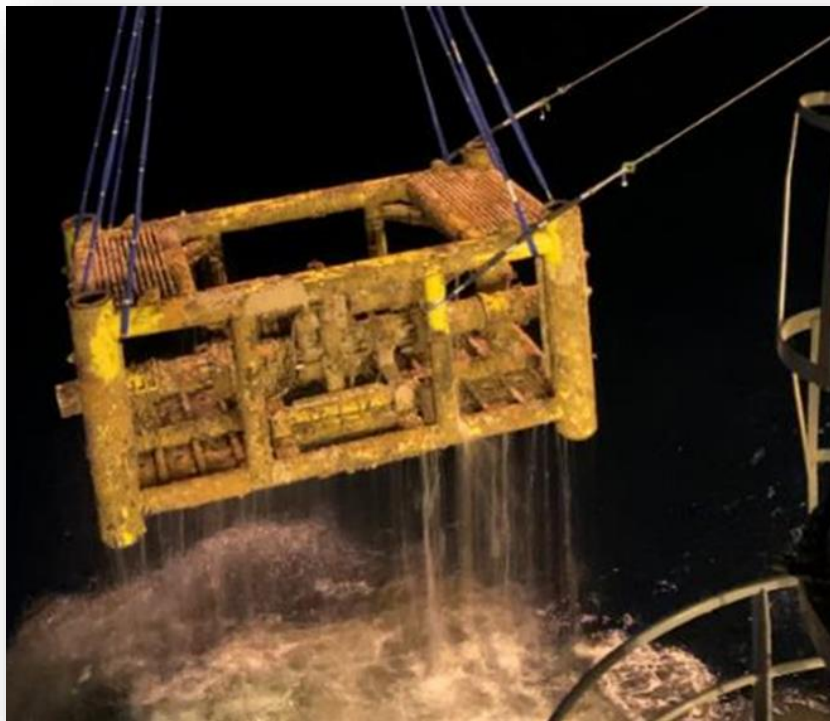
Pipeline subsea isolation valve and associated protection structure
