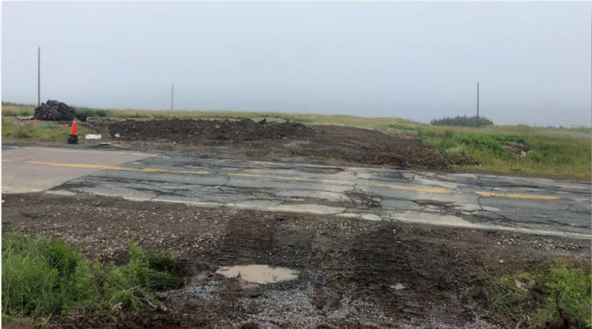
South side (background) of Highway 316 backfilled prior to re-vegetation
