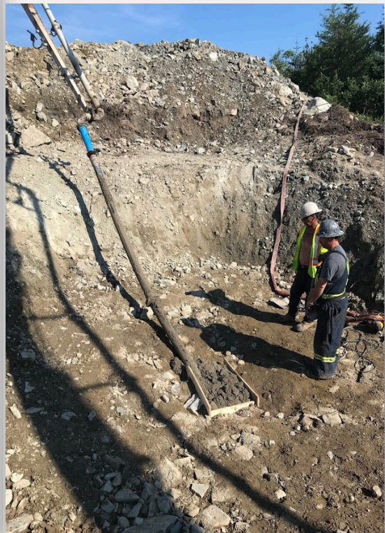
Grouting of the Sable Road crossing
