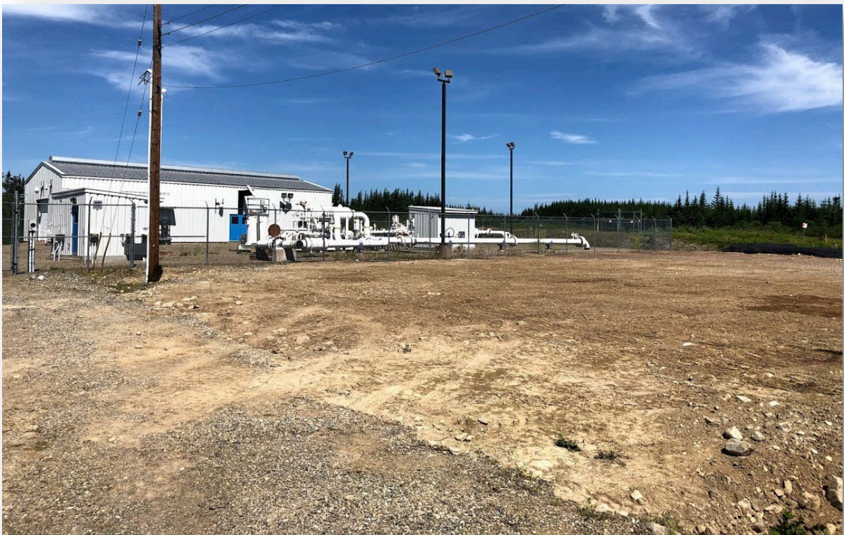
Pipeline terminus infrastructure removal and site grading complete (Maritimes & Northeast Pipeline facilities in the background)
