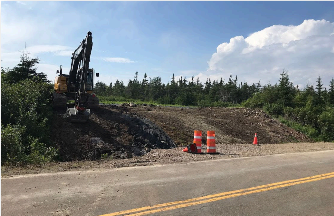
West side of Sable Road backfilled prior to re-vegetation
