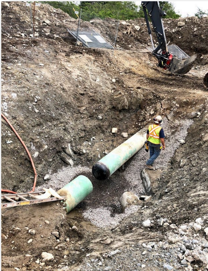
East side of Sable Road, pipeline cap welded
