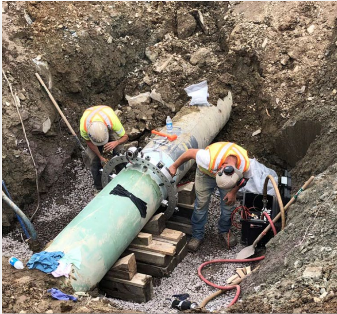
Pipe grouting in progress, north side of Highway 316
