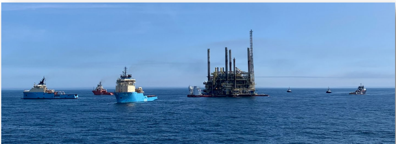
Deep Panuke platform lowered onto Boabarge 34 with legs lifted
