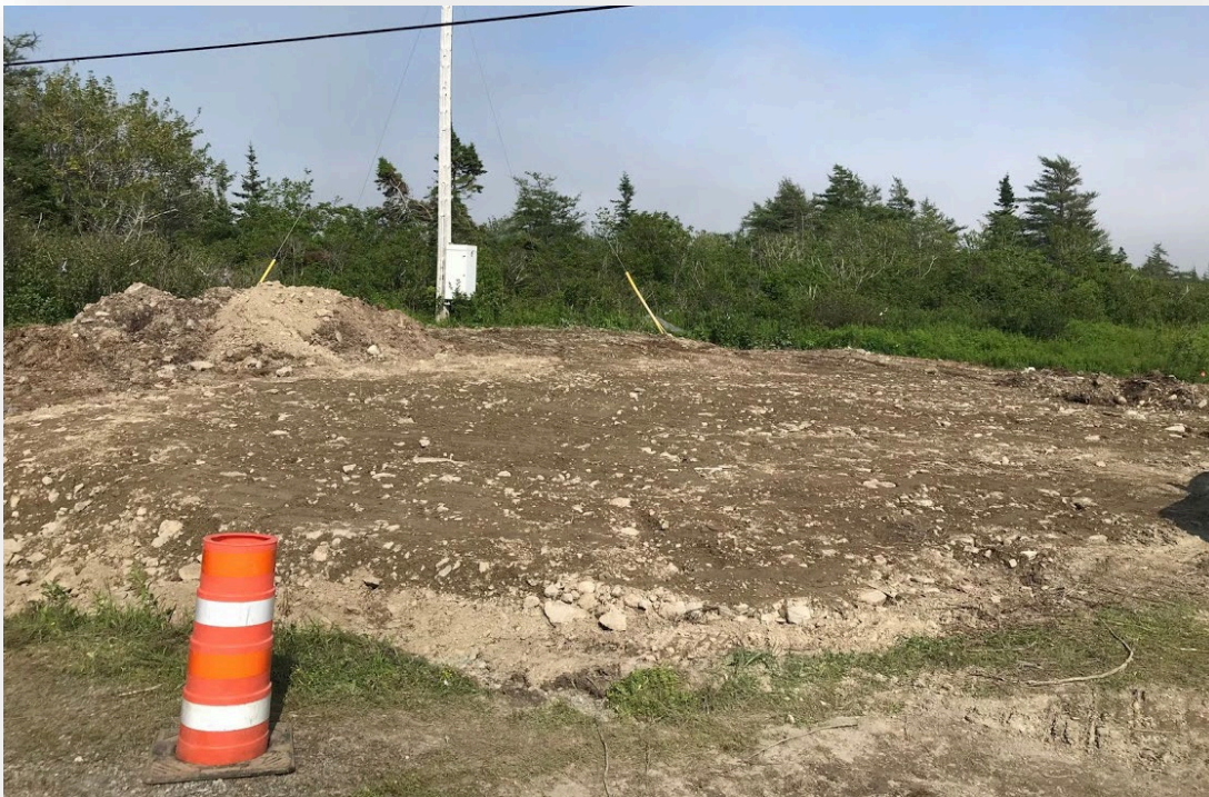
East side of Sable Road backfilled prior to re-vegetation
