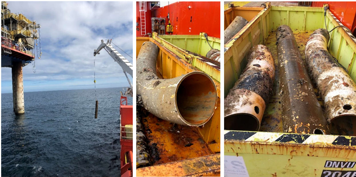
Recovered Sections of Disconnected Pipeline
