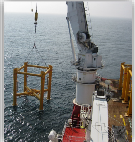
Deep Panuke wellhead protection structure during deployment
