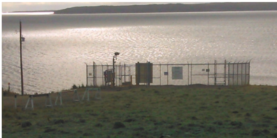
Existing gravel pad, fence and no-anchor sign at the landfall site
