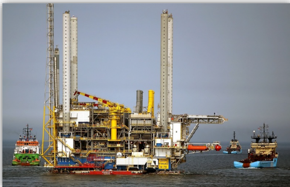
Deep Panuke PFC being towed to site during installation in July 2011
