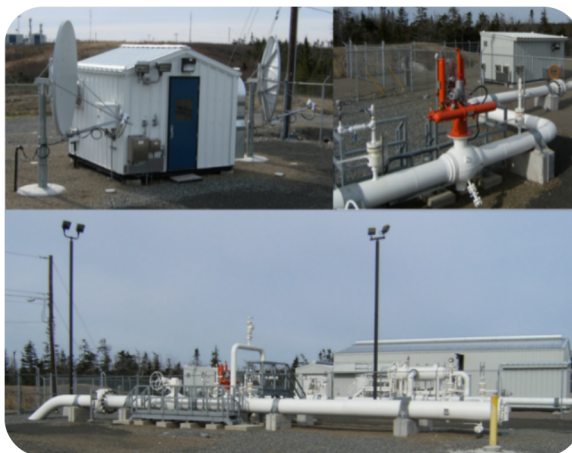
Top left photo: GEP terminus building Top right photo: GEP terminus connection to M&NP Bottom photo: GEP terminus pig receiver
