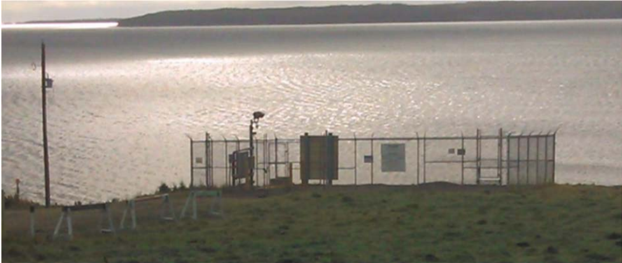
Gravel pad, fence and no-anchor sign at Beach Valve Station before the pipeline flushing program
