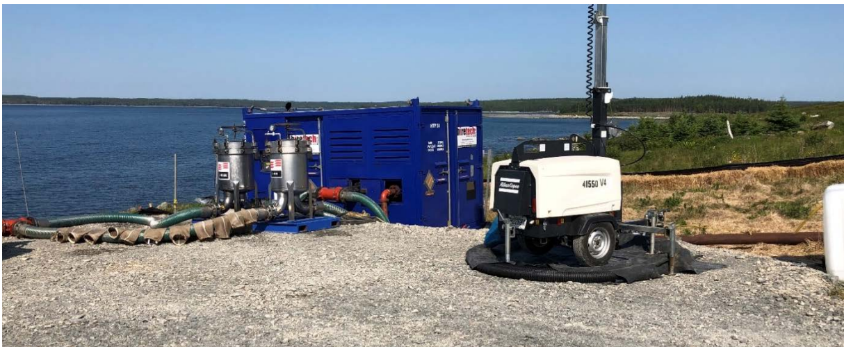
Pumping equipment for the pipeline flushing program at Beach Valve Station
