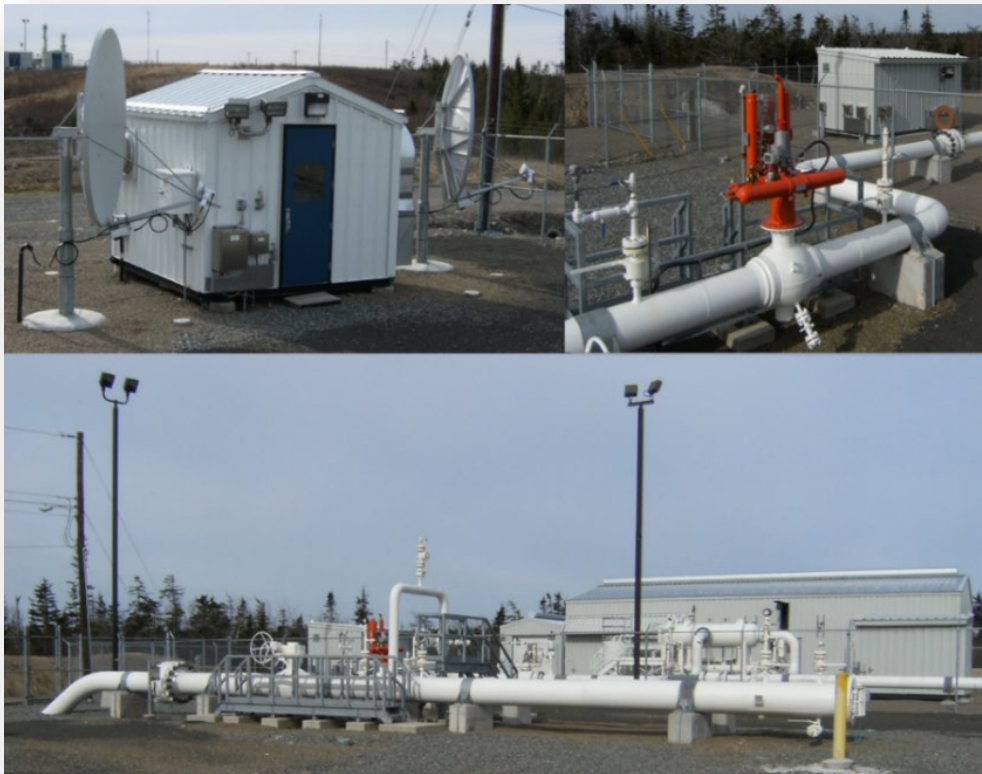
Deep Panuke Gas Pipeline Terminus Facilities near Goldboro, Nova Scotia
