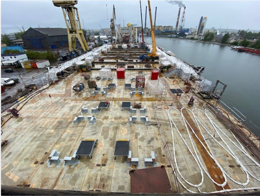
Boabarge 34 Being Outfitted for Platform Deinstallation Operations (May 2020)
